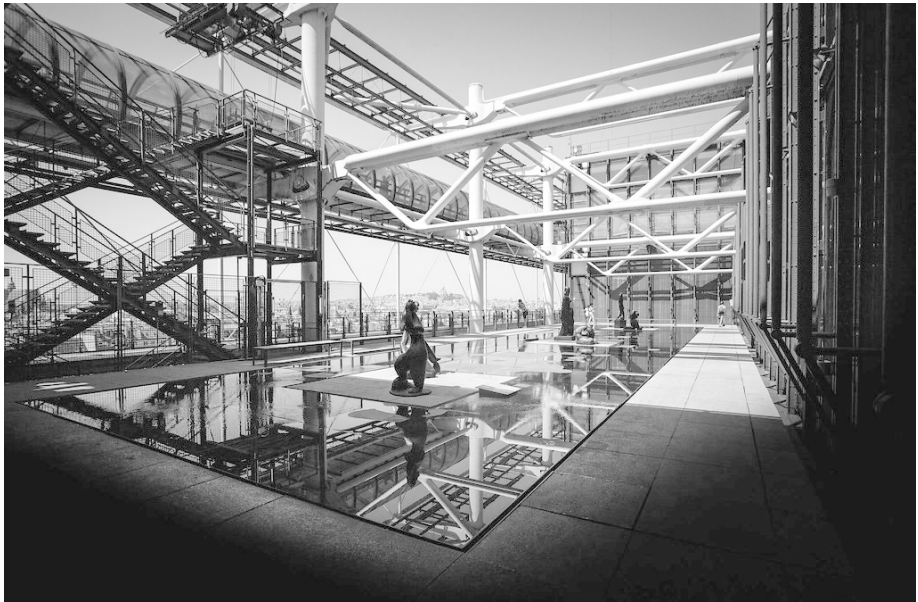
Fig. 2. Beaubourg, or Centre Pompidou, Paris. By Richard Rogers, Sue Rogers, Renzo Piano, and Gianfranco Franchini. Completed in 1977 and rebuilt in 2000.
